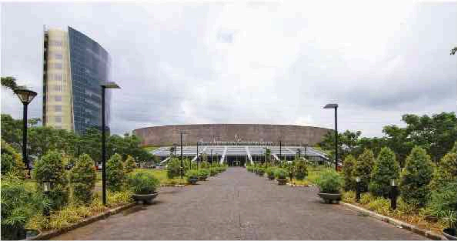
SICC Office Tower
