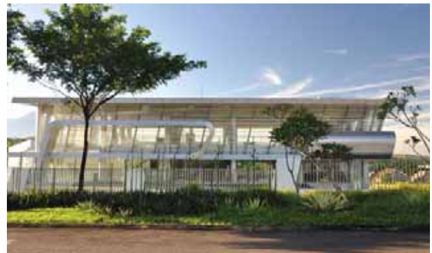
IBM Data Center
