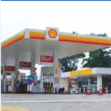
▲ Shell Gas Station
