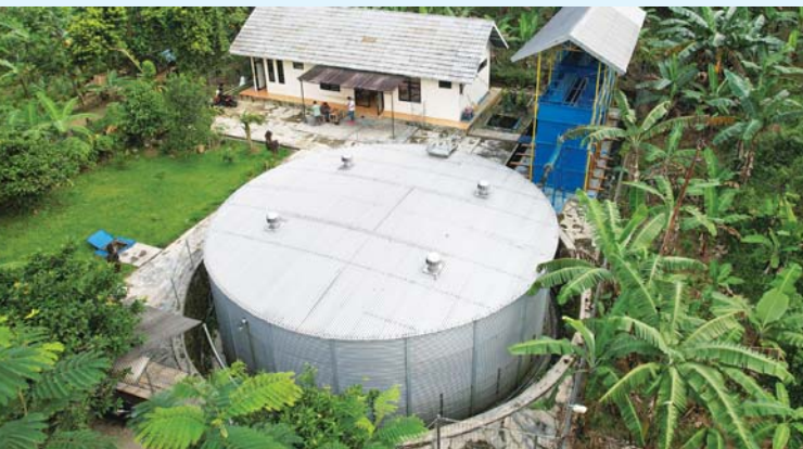
Water Treatment Plant (WTP)
