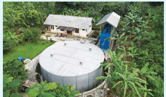
Water Treatment Plant (WTP)
